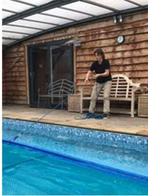
Then walk to the shallow end allowing the rope to play out, pull hand over hand until the cover is flush with the end of the pool before replacing the rope on its hook.
